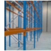
Pallet Racking and Workbenches
